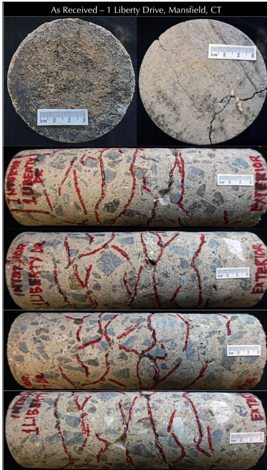
Figure 8: Shown are: (a) the black formed exterior surface of the foundation wall on the core end in the top left photo, (b) smooth, flat, gray formed interior surface of the foundation wall with visible cracks on the core end in the top right photo, and cylindrical side views of the core from 1 Liberty Drive (rest photos), as received, showing full-depth extension of numerous visible cracks due to retrieval of the core from over visible cracks on the wall. Visible cracks on cylindrical surface of core are highlighted, which are mostly concentrated in the interior of the core (wall) than the interior or exterior ends.
