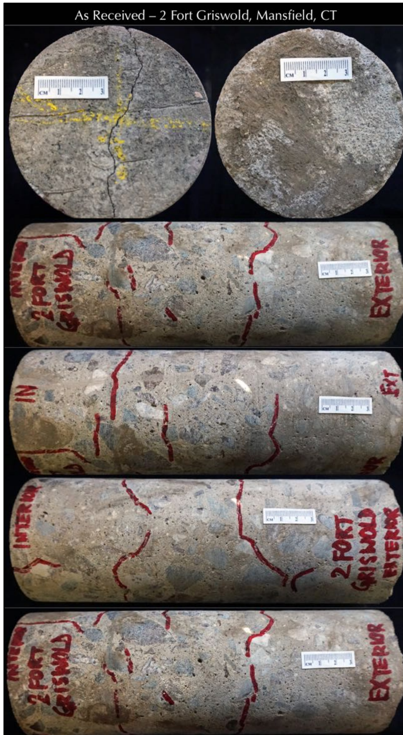
Figure 9: Shown are: (a) the formed exterior surface of the foundation wall on the core end in the top right photo, (b) smooth, flat, gray formed interior surface of the foundation wall with visible cracks on the core end in the top left photo, and cylindrical side views of the core from 2 Fort Griswold (rest photos), as received, showing full-depth extension of numerous visible cracks due to retrieval of the core from over visible cracks on the wall. Visible cracks on cylindrical surface of core are highlighted, which are mostly concentrated in the interior of the core (wall) than the interior or exterior ends. Interior wall has a vertical crack extended to a distance of 1.5 in. inside the core. Notice this core from 2 Fort Griswold residence has less visible cracks in the interior than that from 1 Liberty Drive.
