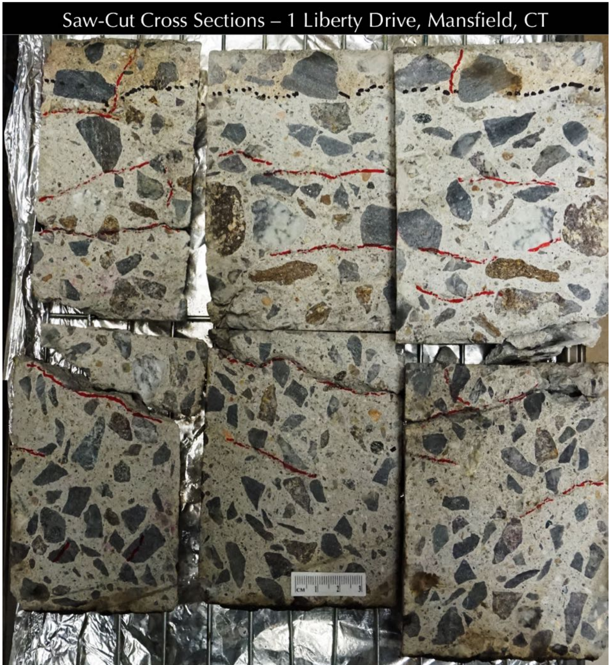
Figure 10: Multiple saw-cut cross sections of the core from 1 Liberty Drive showing: (a) full-depth extension of visible cracks that are highlighted in red (mostly concentrated in the inside of the core); (b) beige discoloration of paste at the interior end of the wall (at the top) and also at the exterior end (bottom) that are marked with black dashed lines at the top, where beige discoloration is due to atmospheric carbonation of concrete during service, mostly occurred along the interior wall surface (to a distance of 20 to 25 mm) than from the exterior end (only 5 mm). Notice a vertical crack from the interior end (at the top) extended to a distance of 1.5 in.
